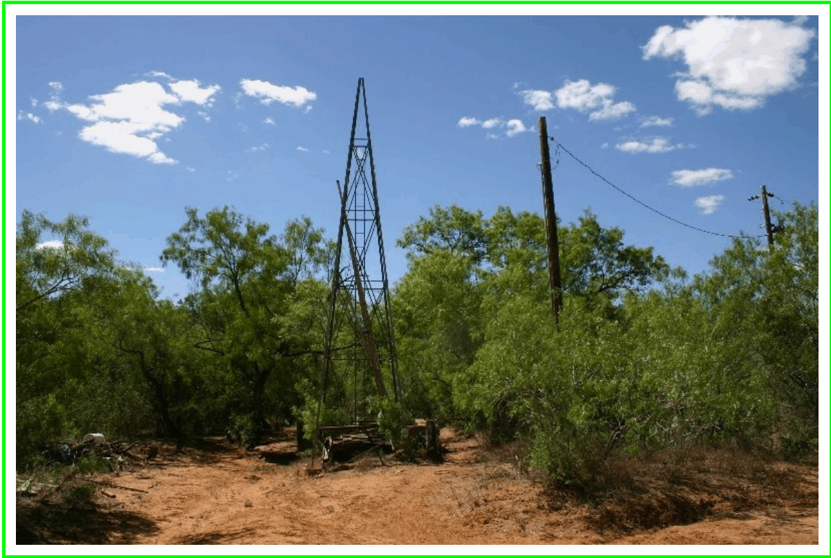
VIEW OF WATER WELL
