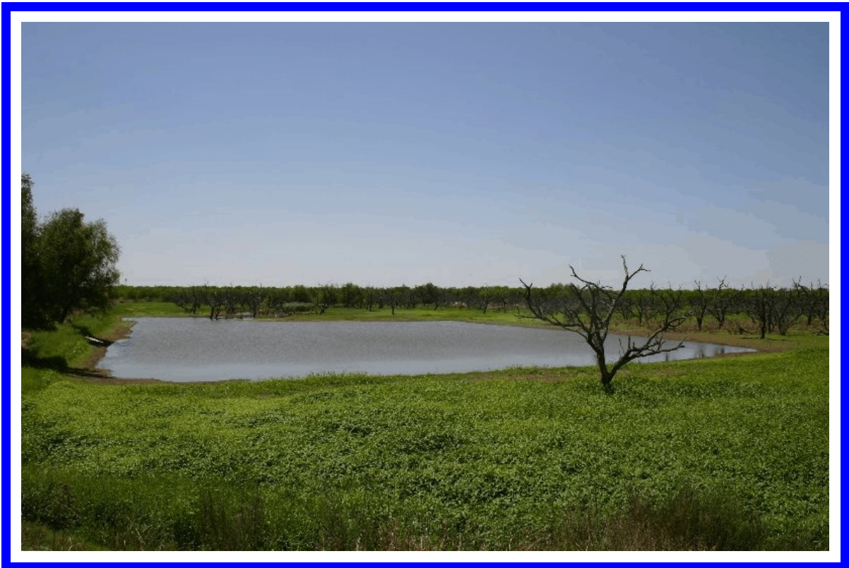
VIEW OF EARTHEN STOCK TANK
